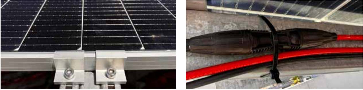
Figure 61: Reinforced with additional end clamps and MC4 connector tie-downs
