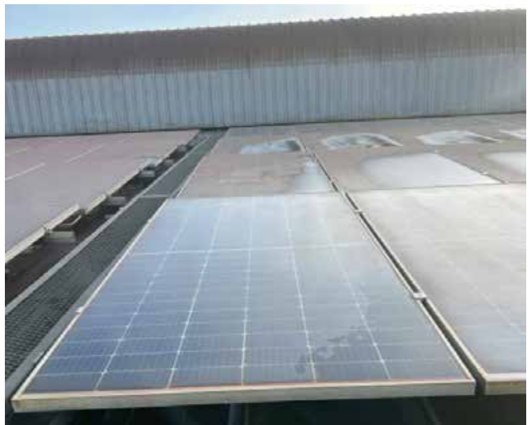
Figure 65: Dust accumulation rates reduce significantly when the PV panels are cleaned with a biodegradable cleaning chemical
