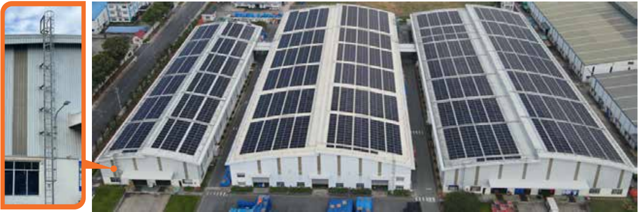
Figure 56: Location of access to the roof and ladder to the roof
