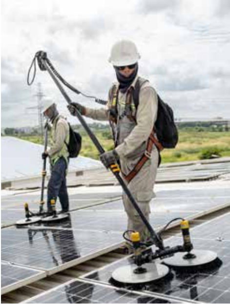
Figure 27: Cleaning PV panels
