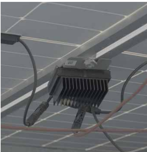
Figure 35: DC Optimiser installed under a PV panel
