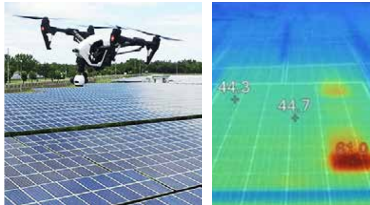
Figure 34. Detecting faults in PV panels using drone with thermal sensors
