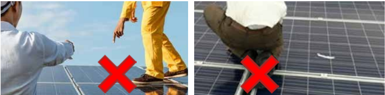
Figure 31: Do not climb, sit, or stand on PV panels
