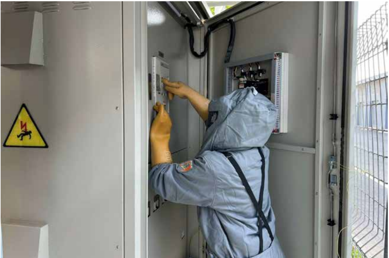
Figure 49: Technician performing on-site repairs
